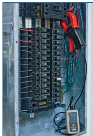
L101 recording branch circuit current.
